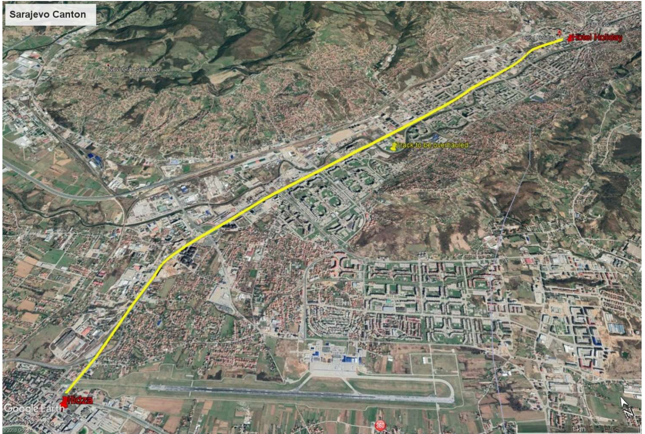
Figure 1 - Tram railway reconstruction
